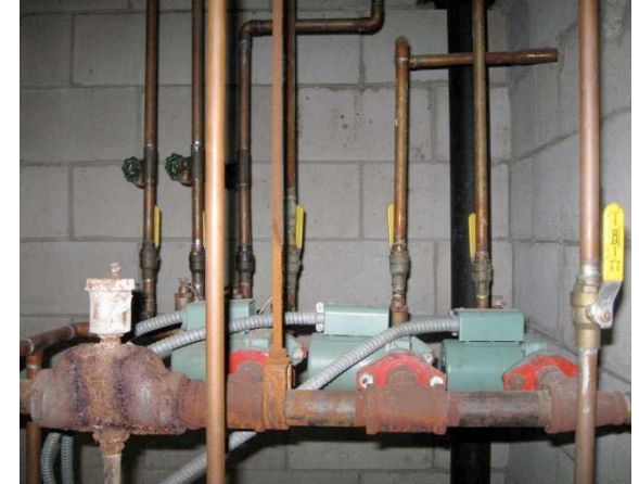
#4— Pipes over boiler before (above) and after (below). Insulate heating and DHW pipes in non-occupied spaces. Get heat and domestic hot water where the people are!
