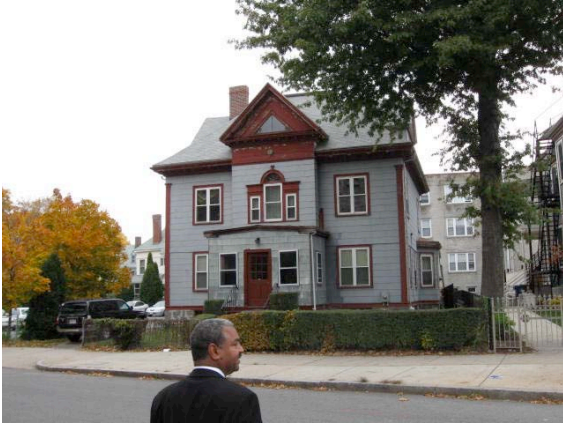
#1 — 5 Elm Hill Avenue is a 3 story + basement building, providing office, meeting and residential space.
