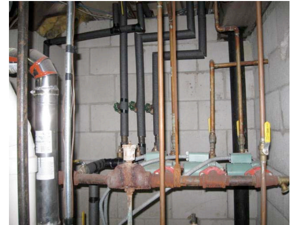
#4— Pipes over boiler before (above) and after (below). Insulate heating and DHW pipes in non-occupied spaces. Get heat and domestic hot water where the people are!
