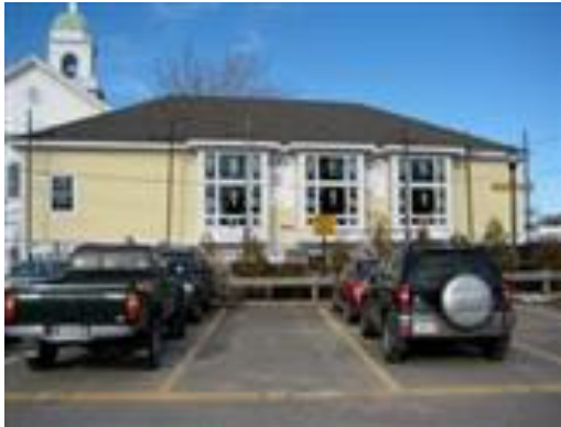
The congregation is able to share an adjacent parking lot with the town of Needham, so no additional impervious surface was created; site gardens were retained. South-facing windows provide natural heating via solar gain in winter.
