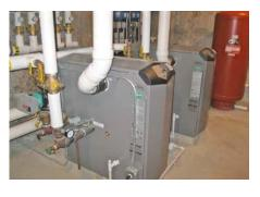
95±% efficient gas-fired condensing mode hydronic boilers, shown at right.
