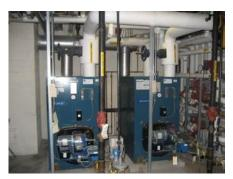
Temple Beth Shalom in Needham has made efforts in recent years to reduce energy bills and carbon footprint. In 2003, Beth Shalom switched from a low efficiency oil furnace to two gas---fired hydronic boilers that have 88% efficiency. (See photo at left.) At \$1.60 per gallon of oil compared to \$1.30 per therm, the new Burnham systems save the Temple \$3---\$4,000 every year.
