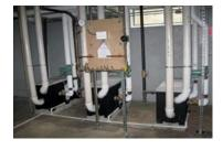
Three high efficiency (93%+) gas---fired condensing mode boilers were installed, with digital controls including one that senses outside temperature. The three boilers permit rotation, extending the life of all boilers and ensuring that the building is never without heat because of boiler failure. The boilers serve several zones, each separately controlled.
