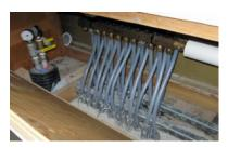
The Sanctuary was cleared, with the placement of pews carefully plotted for replacement without penetrating any new radiation piping. Old concrete was removed. New "plastic" piping installed with distribution
