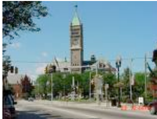
Lowell City Hall 375 Merrimack St. Lowell, Massachusetts
