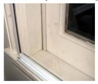
My first window was a hybrid: *magnetic strip* for the sides and top, and a *plastic extrusion* for the bottom, which fits flat on top of a window sill (See diagram 1.) Works well, looks good, but somewhat expensive and time-consuming to build.
